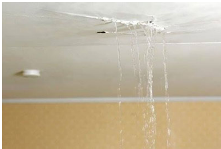
Water penetrating when it rains
