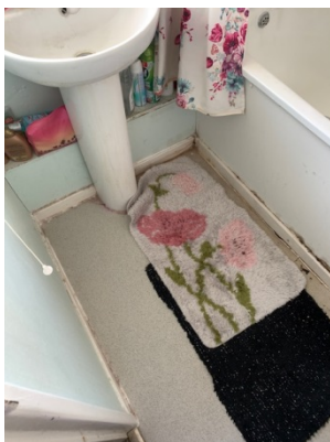
Poor seal to bathroom floor perimeter, allowing water to penetrate leading to wood rot.
