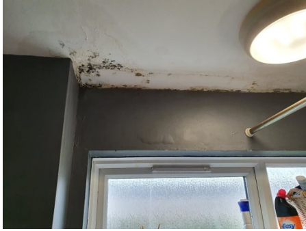
Obvious internal water damage
