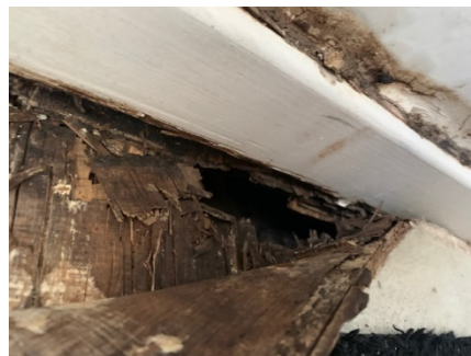
Poor seal to bathroom floor perimeter, allowing water to penetrate leading to wood rot.
